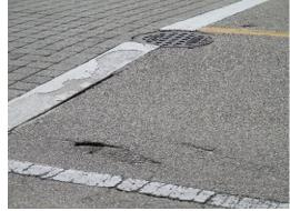
c. Gutters: Gutter pan cracking in front of 3757 and 3761 Buttonwood way was observed. Recommend we contact vendor for repair proposals.
